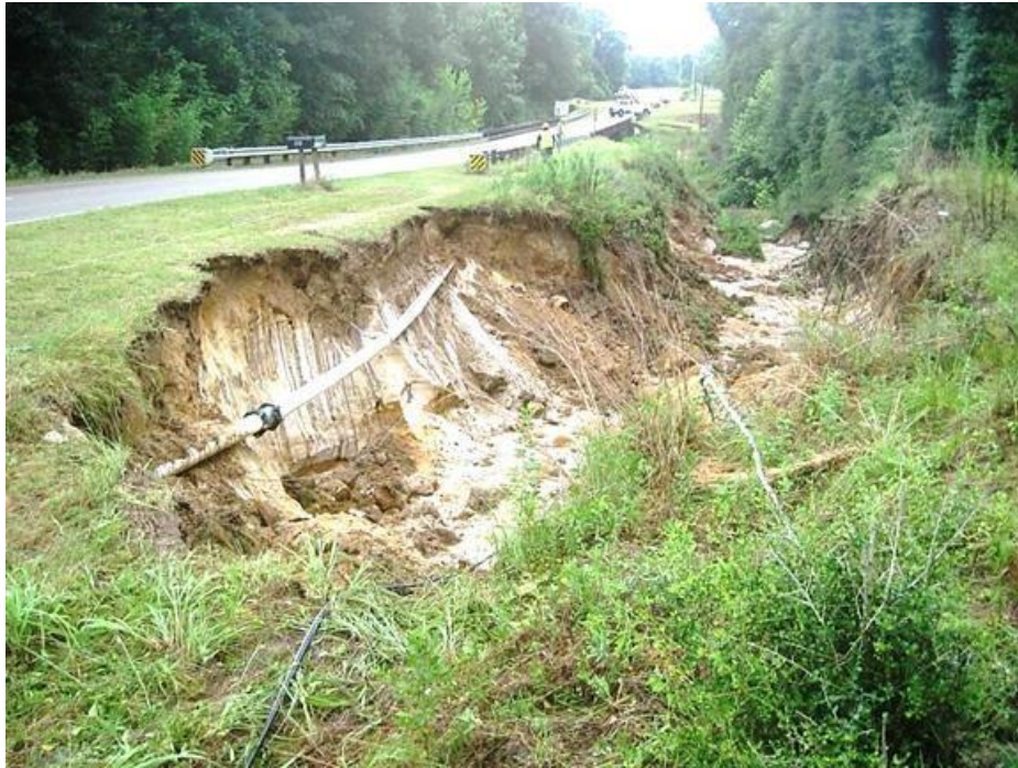
Figure 6. Bed incision in the main channel has triggered a valley trench gully up the side of this road, Alabama. Note exposed utility pipeline.
